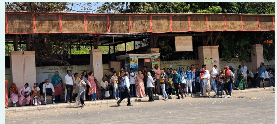
A bus stop in Ahmedabad, India with high-pressure misting systems drop ambient temperatures by 6 - 7°C and traditional vetiver grass and straw curtains naturally regulate heat and provide shade. Source: Mahila Housing Trust.
