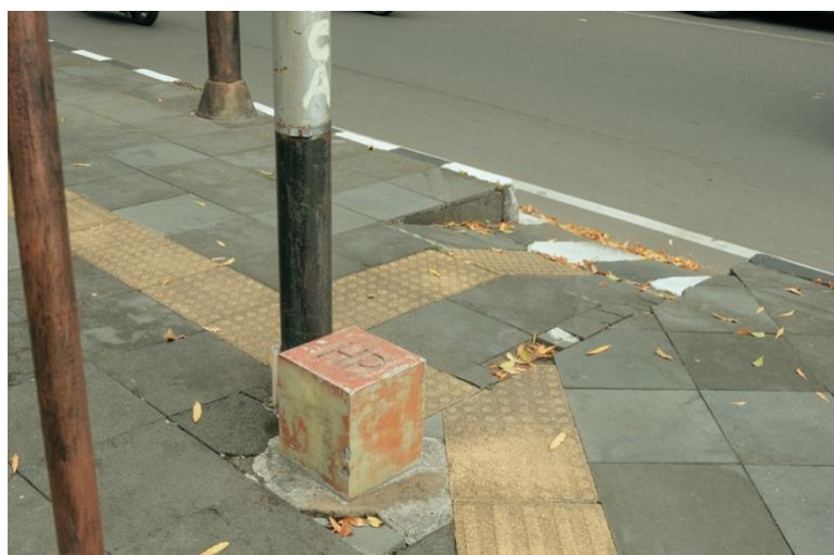
Mis-construction of guiding block paving in the City Walk (Slamet Riyadi St.)
