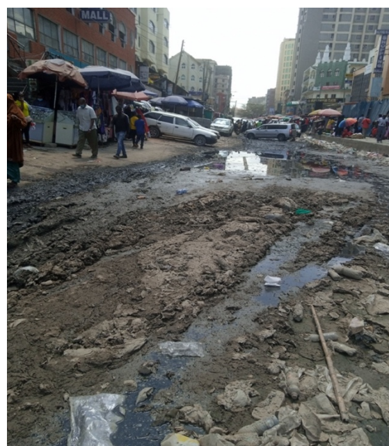
Example of flooded road
