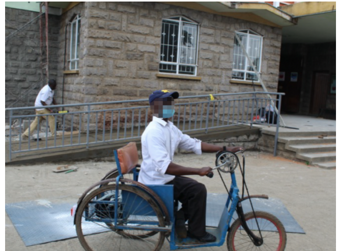
Example of accessible ramp at place of worship
