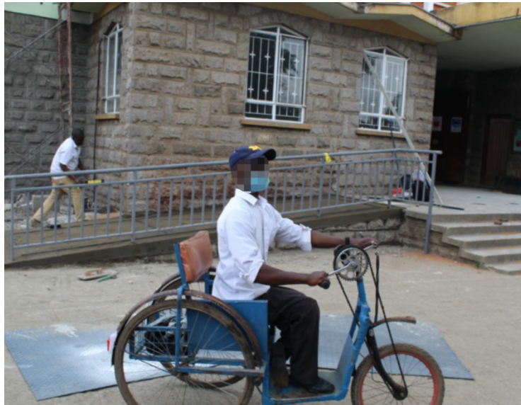
Example of accessible ramp at place of worship
