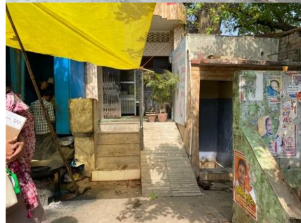
Examples of inclusive design interventions that are not fit for purpose and do not meet standards.
